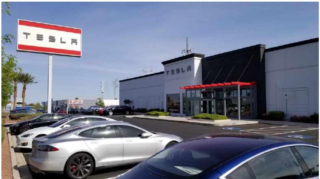
PHOTO – Tesla opened a 26,000-square-foot sales and service store at 7077 West Sahara Avenue in early 2018. The showroom displays the company's energy products and test drives are available by appointment. There are two supercharger stations and multiple destination chargers located throughout the valley.
