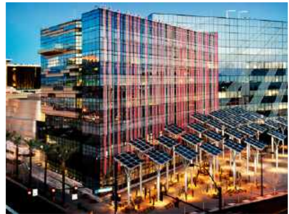
PHOTO – Located at 495 S. Main Street, City Hall is an energy-efficient structure that is built to LEED® standards, reducing energy costs by more than $500,000 annually. Photo by Ryan Reason.
